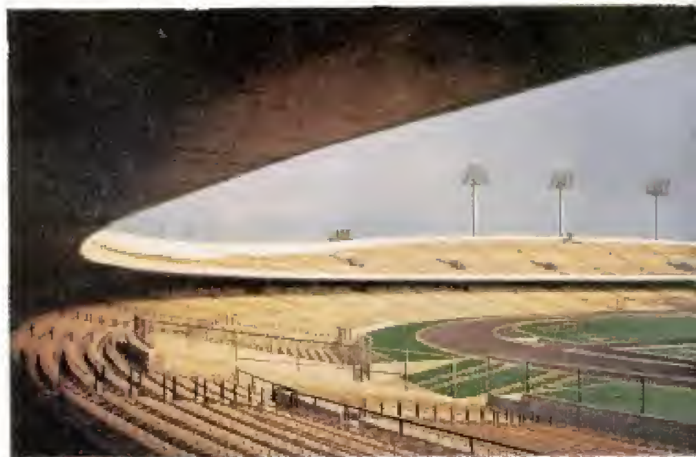
Seating areas are reached through 48 tunnels. Running track of the stadium is surfaced in black volcanic crushed rock. Below, three swimming pools are interconnected so casual swimmers can wander from one to another. Underwater windows help the coaches train their student swimmers
